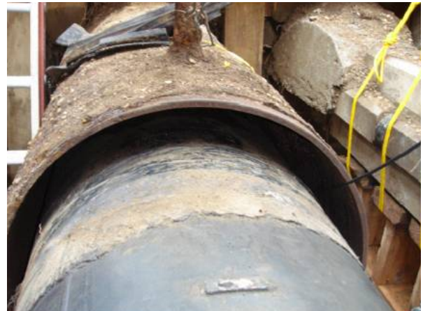
Figure 1: Cased Pipe Exposed for Test
