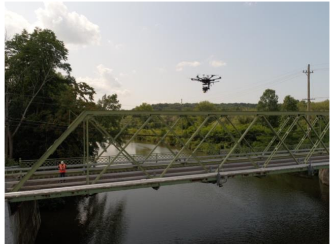
Figure 1: Performing leak detection with a sUAS mounted methane sensors
