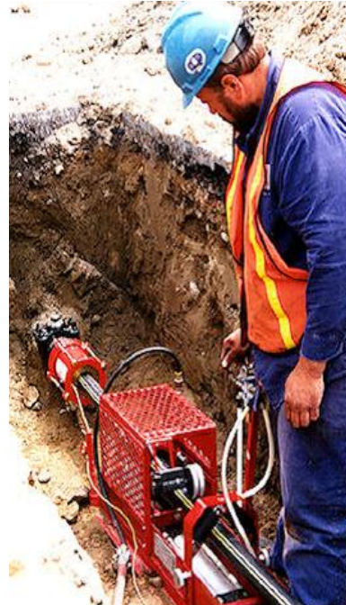
Figure 2: Live Main Insertion Demo
