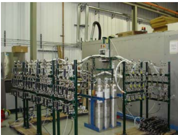
Figure 1: Testing Setup with Environmental Chamber in the Background
