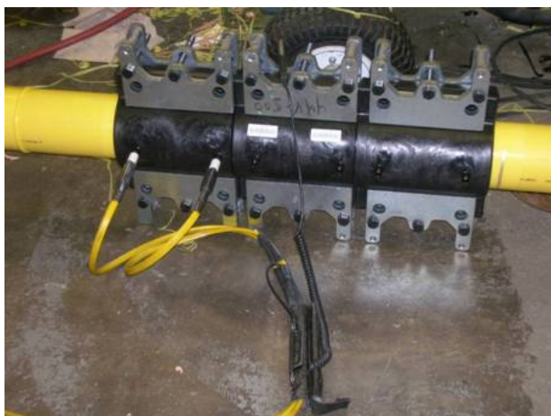
Figure 2: VLRS Electrofusion Process
