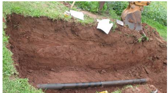
Figure 1: Exposed Pipe as Part of Integrity Assessment
