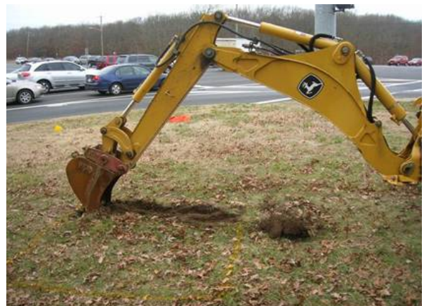
Figure 2: Typical Backhoe Excavation
