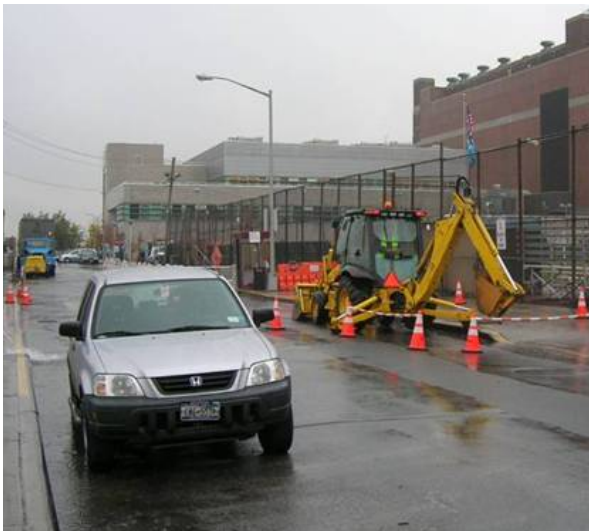
Figure 2: Backhoe Excavation — Urban Site
