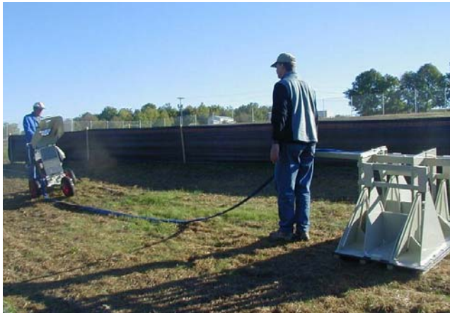
Figure 2: No-Pig Above Ground Inspection
