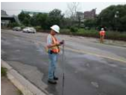
Close Interval Survey Measurements being taken as part of DA Process
