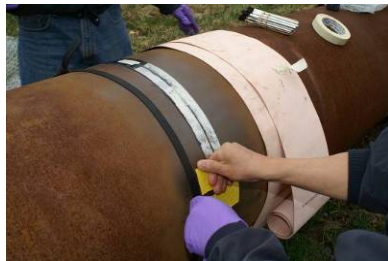
Installation of the Magnetostrictive Strip
