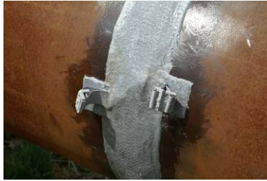
Complete MsS Installed
