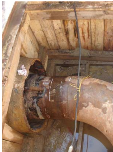
30" Carrier within a 48" Cast Iron Casing
