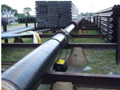
ConEdison Astoria Yard Field Mockup
