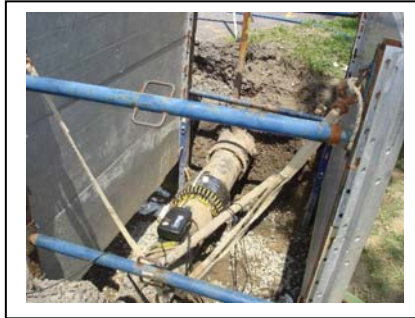
Sample cased crossing exposed with shoring
