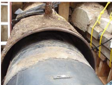
Cased Pipe Exposed for Test
