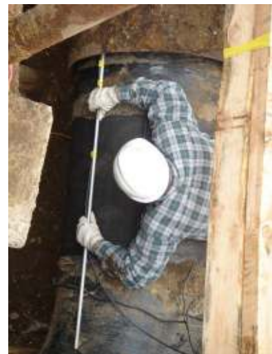
Pushrod Mounted Camera In Use
