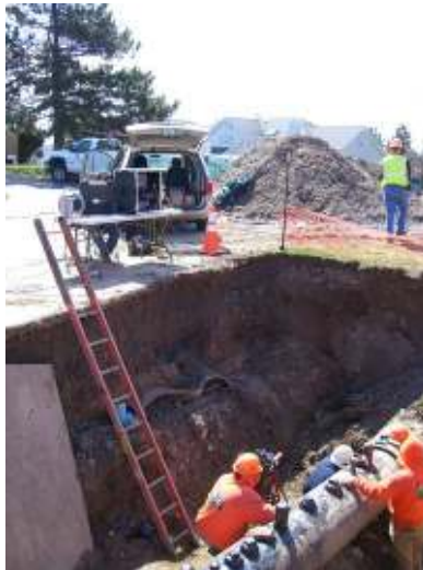
Field Testing an 80' Section of a 24" Carrier within a 30" Casing
