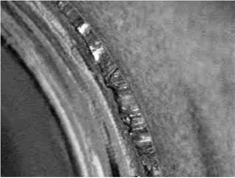
Inspection of welded joint
